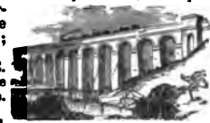
Viaduct of Masonry.
